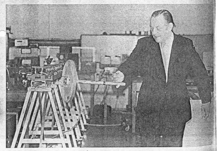
Fig. 5.-A 24 lb gyro rising from the action of a little finger
